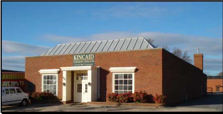
Stand-alone Kincaid Furniture building – almost 6,000 sq. ft. with plenty of parking – perfect for branch bank or restaurant!
